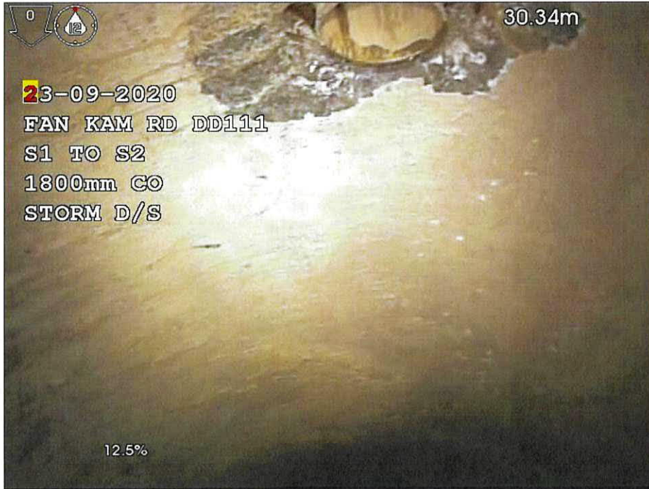
Photo Ref. : 005 Video Tape : 0001, 0:03:09 Observation : Connection, at 12 o'clock, dia 150 mm
